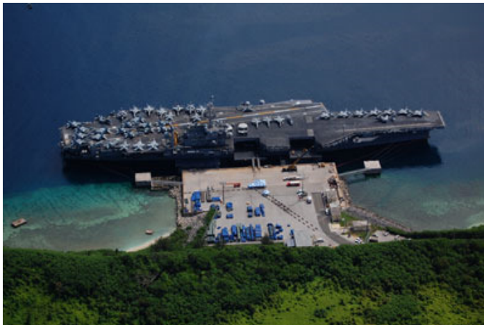
Guam's military build-up includes a new wharf for aircraft carriers.
